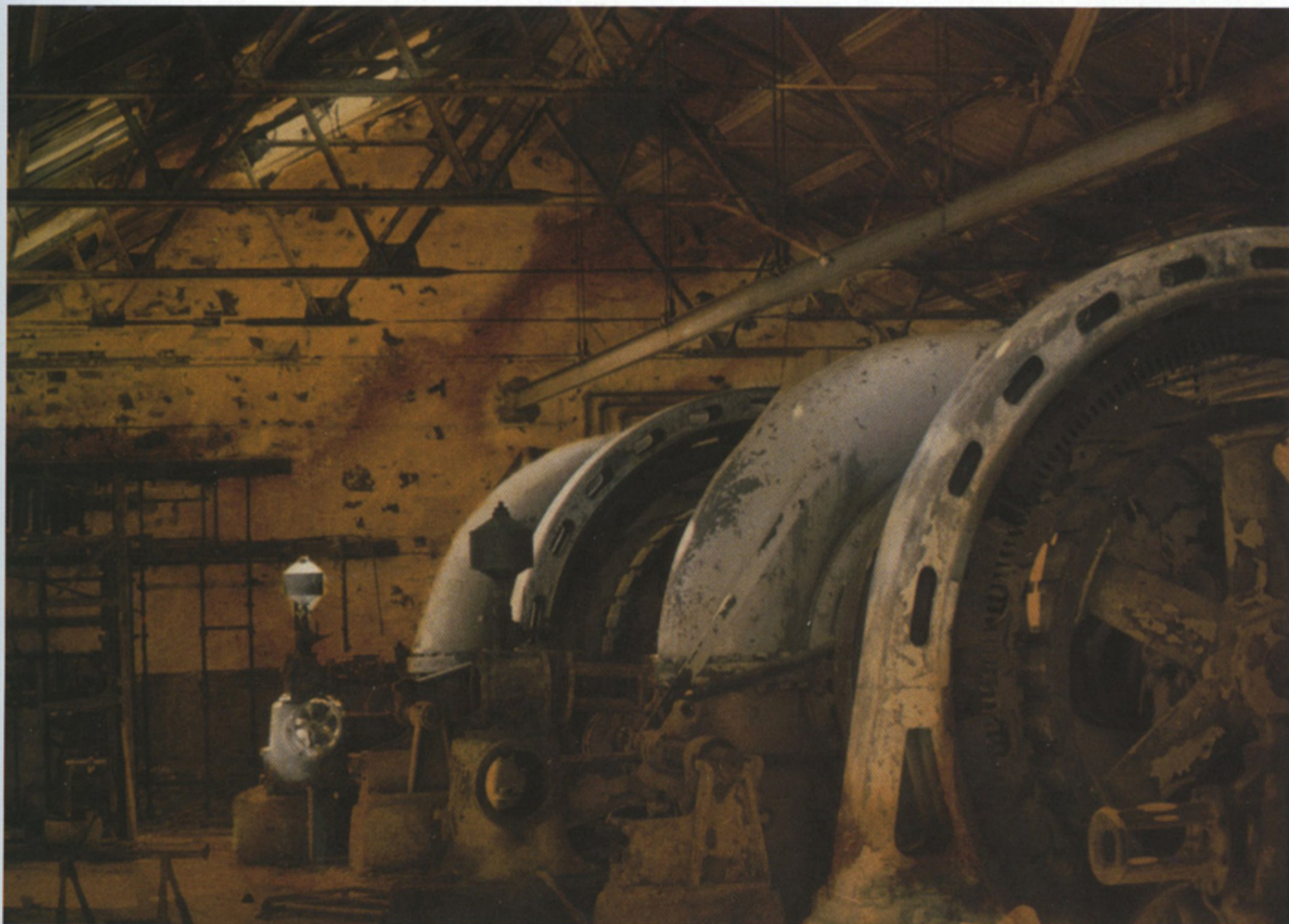
Power House, White River, Oregon, 1996
